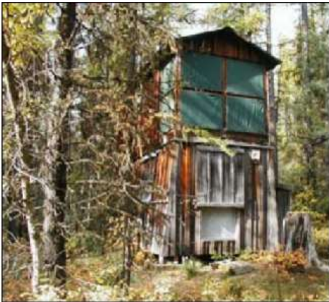
The only cabin in the subdivision in 2002. Photo by Lloyd Barrie of Barrie Appraisal
