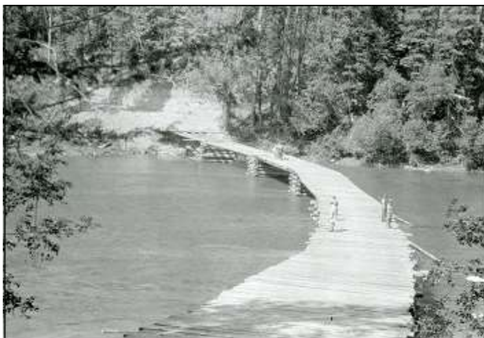
A photo of the bridge the Lee Brothers built across the Middle Fork to log their property in Glacier National Park. Courtesy of Arne Boveng
